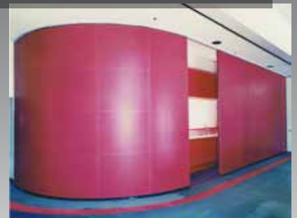
SAN DIEGO CONVENTION CENTER, SAN DIEGO, CALIFORNIA Curved panels and track. Perforated sound absorptive panel faces, NRC 0.65, manual operation.
