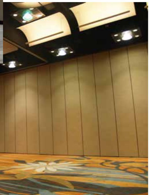
HOTEL GRAND HYATT MACAU CITY OF DREAMS, CHINA ALPHA 'S' panel, welded steel construction, 16 gauge steel faces, manual operation. Height 26' - 3" (8 meters). Architect: HBA Design Consultants Installed: 2013
