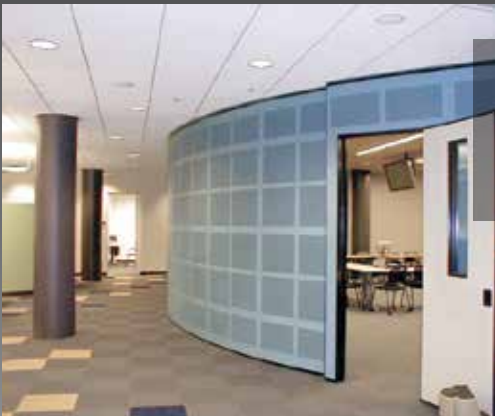
G.E. CAPITAL, UNIVERSITY OF CONNECTICUT, STORRS, CONNECTICUT Bi-parting, electrically operated, curved panels and track with four panel elements traveling on two parallel tracks. Perforated sound absorptive panel faces with paint finish, inset pass door with lite also by AEC. Architect: CPG Architects and Planners
